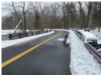
Folly Lane Bridge is substantially complete and has reopened for the winter. Some temporary closures will be required in the spring for final paving.
